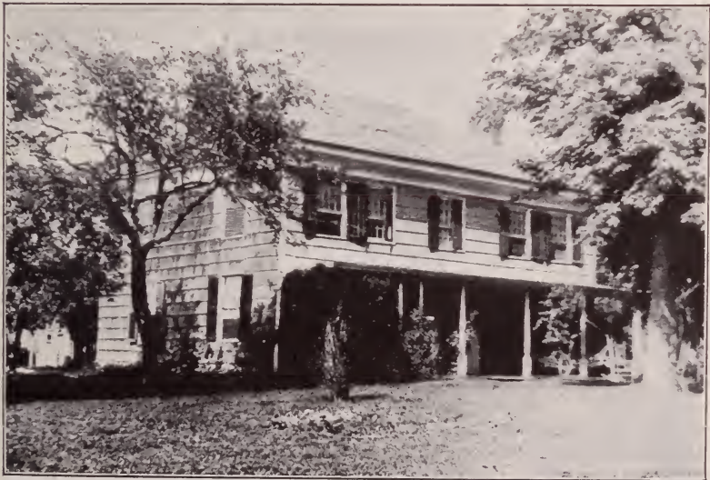
THE BUDD—BRADDICK HOUSE, SOUTHOLD, L. I. (Photographed specially for this work)
